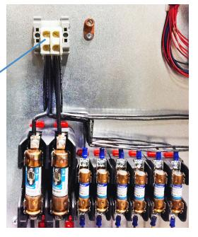
Some chiller manufacturers have multiple connection requirements before all power needs and functions are operational. All Legacy chillers come <u>standard</u> with **One Single Point Power Connection** for all functions and operations.
