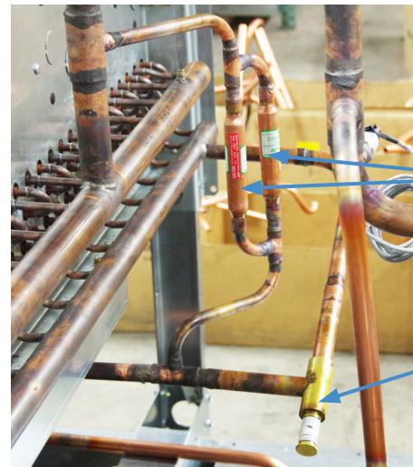
Installed - Head Pressure Control Valve (adjustable for larger chillers)
