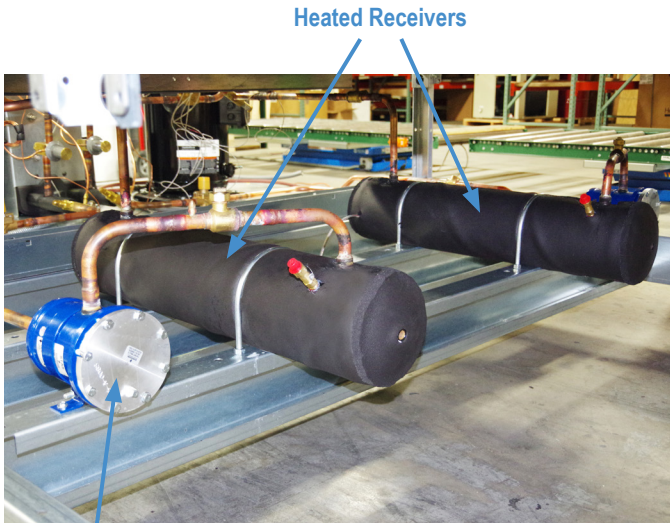
Installed - Heated Receivers
